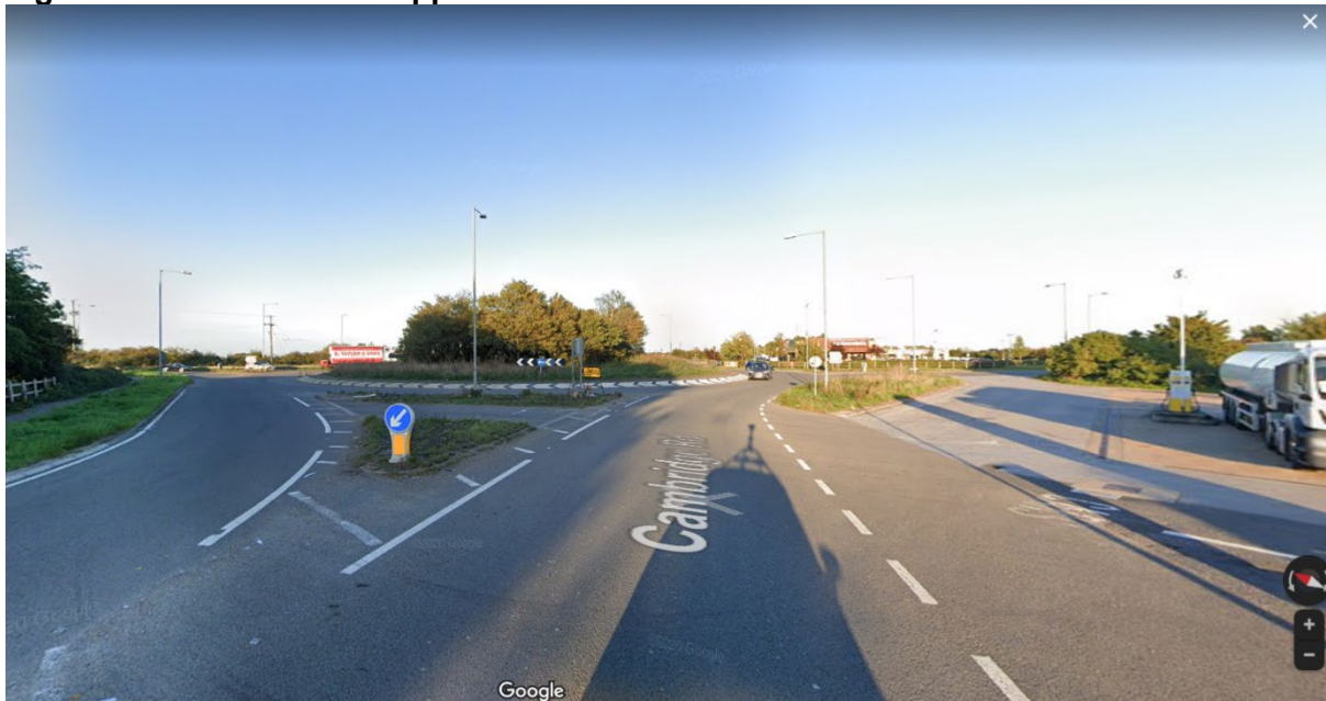
Figure 2E A428 West Approach to Caxton Gibbet Roundabout
